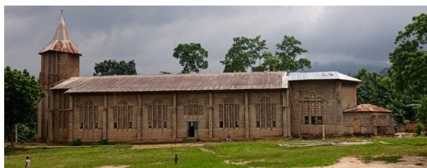
Our Lady of Lourdes Parish, with its new choir roof on the right and the bell tower on the left.
